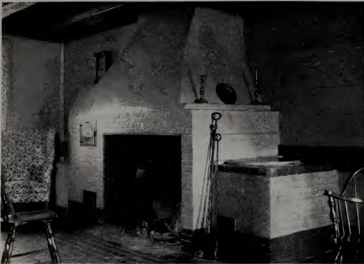
Moor Russell's kitchen of 1797, equipped with a fireplace with an iron kettle on the crane, the brick oven, and an iron kettle enclosed with bricks and with a fire box beneath it. The family of four people lived in this room several years.
